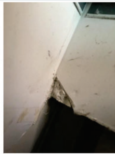
PHOTO 2 | Drywall Joint Compound Atrium Non-ACM
