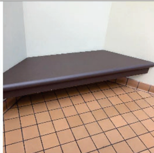
PHOTO 2 Brown Painted Bench < 0.5% lead (by weight)
