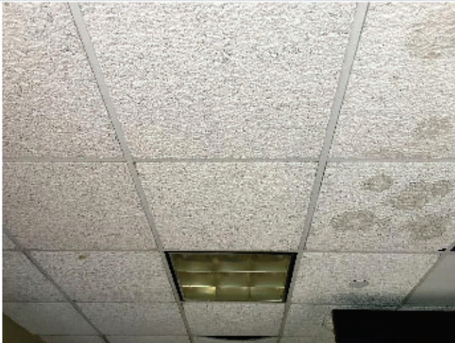
PHOTO 1 | 2' x 2' Ceiling Tile Entry Non-ACM
