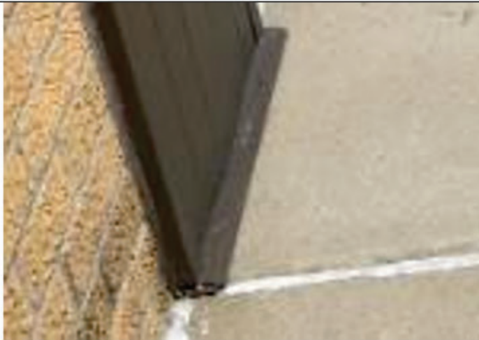
PHOTO 9 Black Exterior Base Caulk Non-ACM
