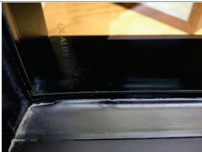
PHOTO 5 | Black Caulk Interior Windows Atrium Non-ACM
