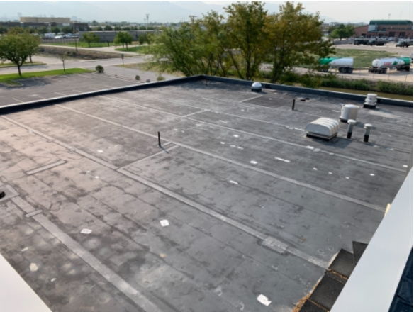
View of Lower EPDM Roof
