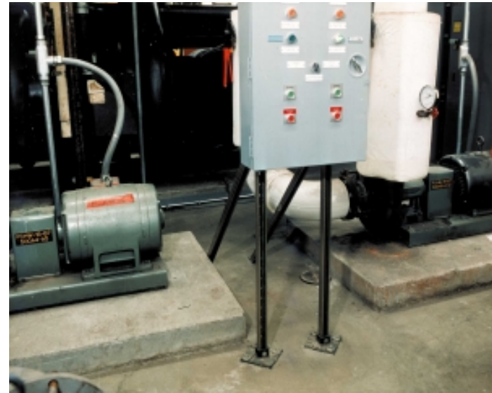
Figure 156: Typical control panel support using angles. Additional angle supports may be required (see below).
