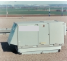
Figure 11: Small rooftop air handling unit.
