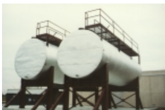
Figure 60: Horizontal tanks including concrete-lined tanks.
