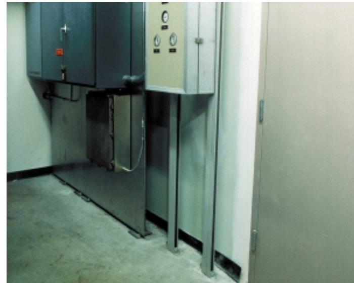
Figure 157: Two different ways to support control panels: using a metal plate attached to floor and ceiling with steel angles (left); using struts extending to floor and ceiling (right).
