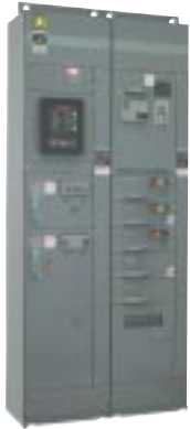
Figure 38: Low voltage motor control center (floor-mounted).
