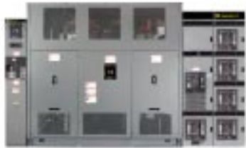
Figure 25: Substation (floor-mounted).
