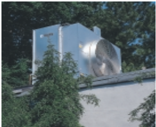
Figure 36: Fluid cooler cross flow with self-contained sump.
