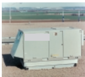
Figure 11: Small rooftop air handling unit.
