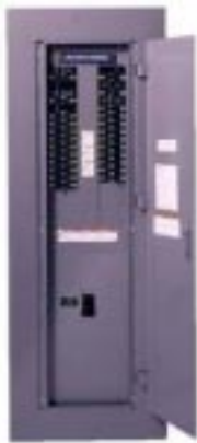
Figure 22: Panelboard (flush wall-mounted).
