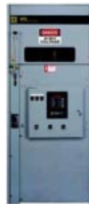
Figure 31: High voltage circuit interrupter (floor-mounted).
