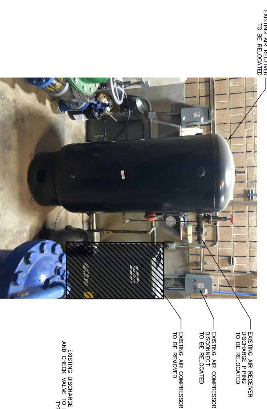
P1 PHOTO 1 - SOUTH WALL RELOCATIONS d1p2
