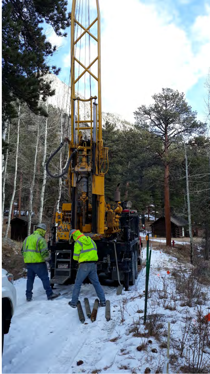
Figure A 6. Drilling boring YA-NW-1.
