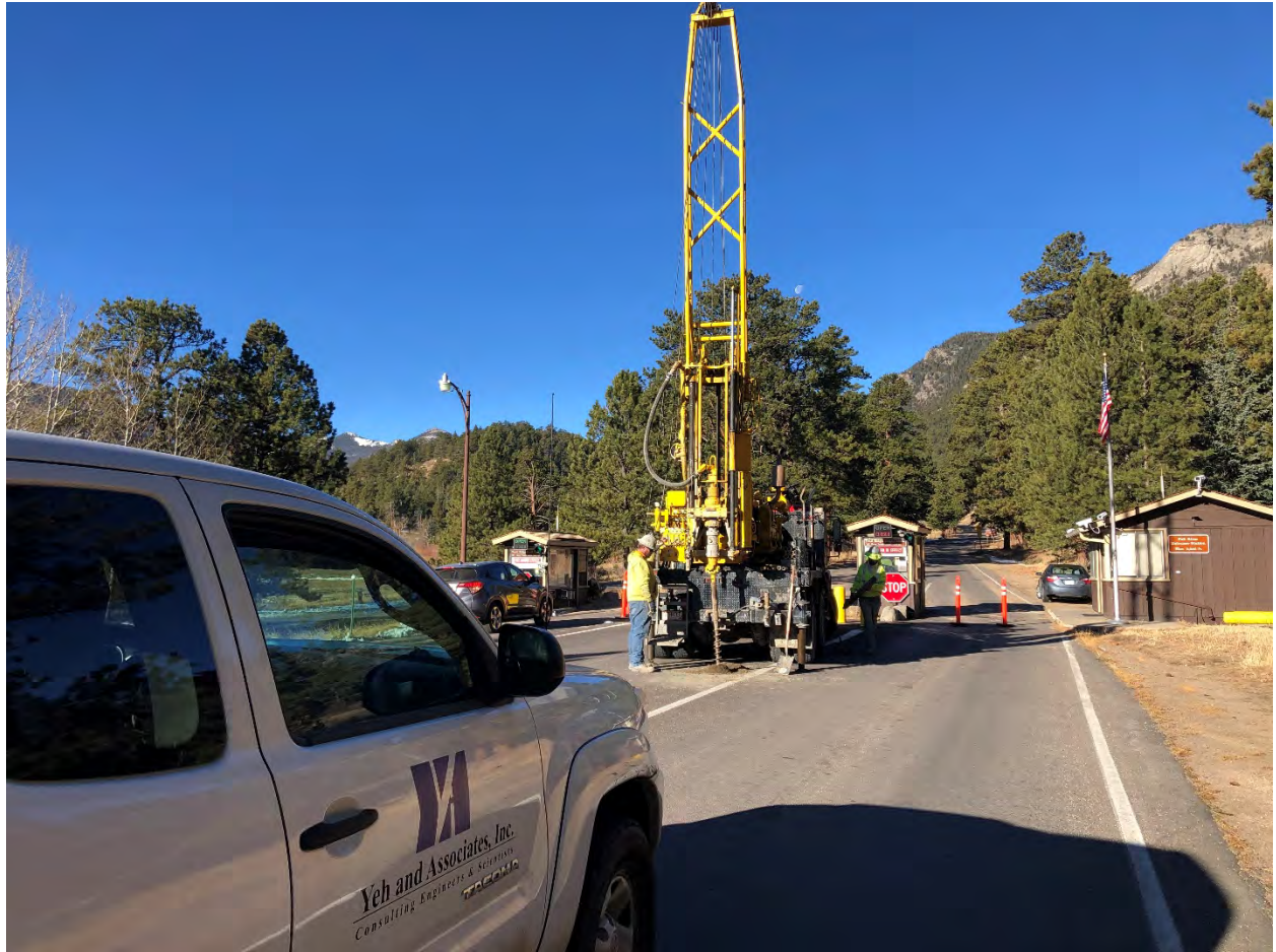
Figure A 7. Drilling boring YA-K1.
