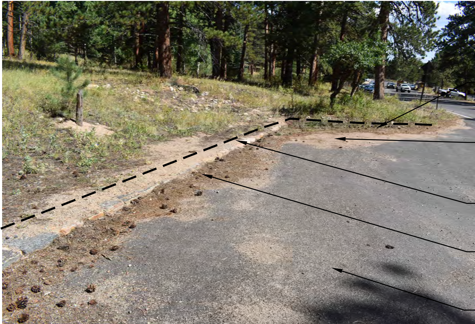
NORTH STONE CURB (LOOKING EAST) — REPAIR
