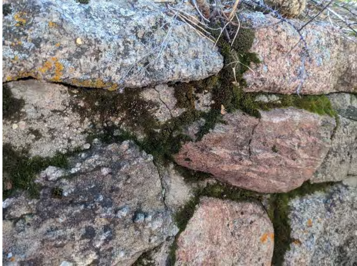
Example photograph of historic stone in Bighorn Ranger Station culvert headwall.
