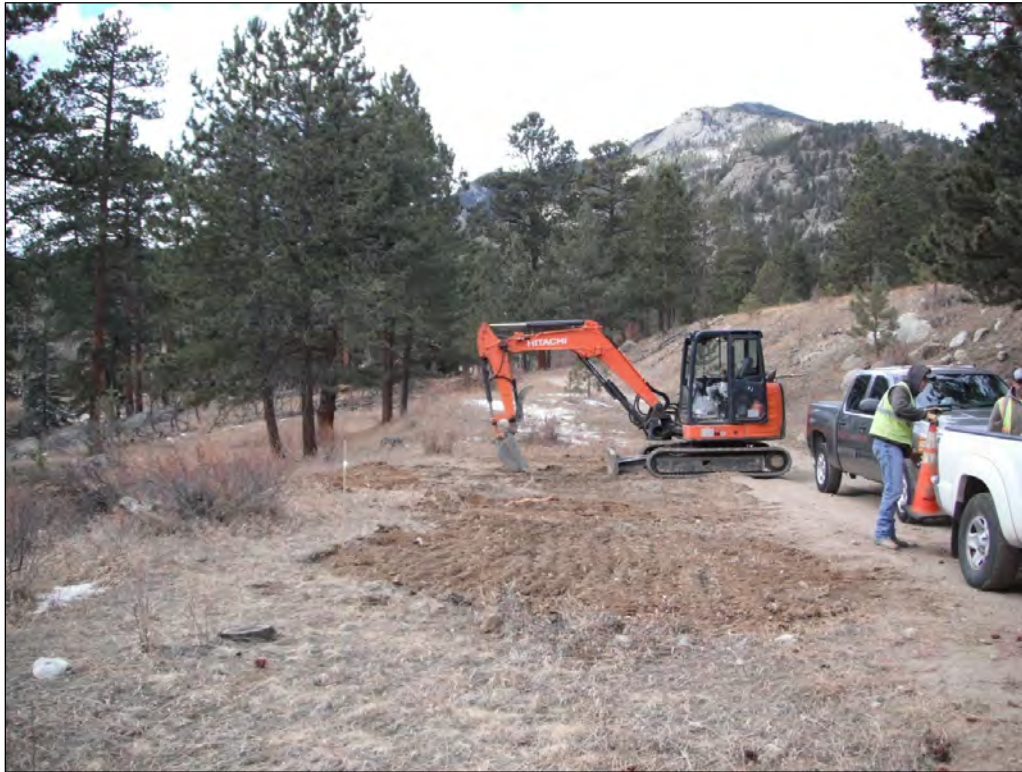
Figure 2. Overview of monitoring area, view to the west. (Photo roll 20-866, image 15)
