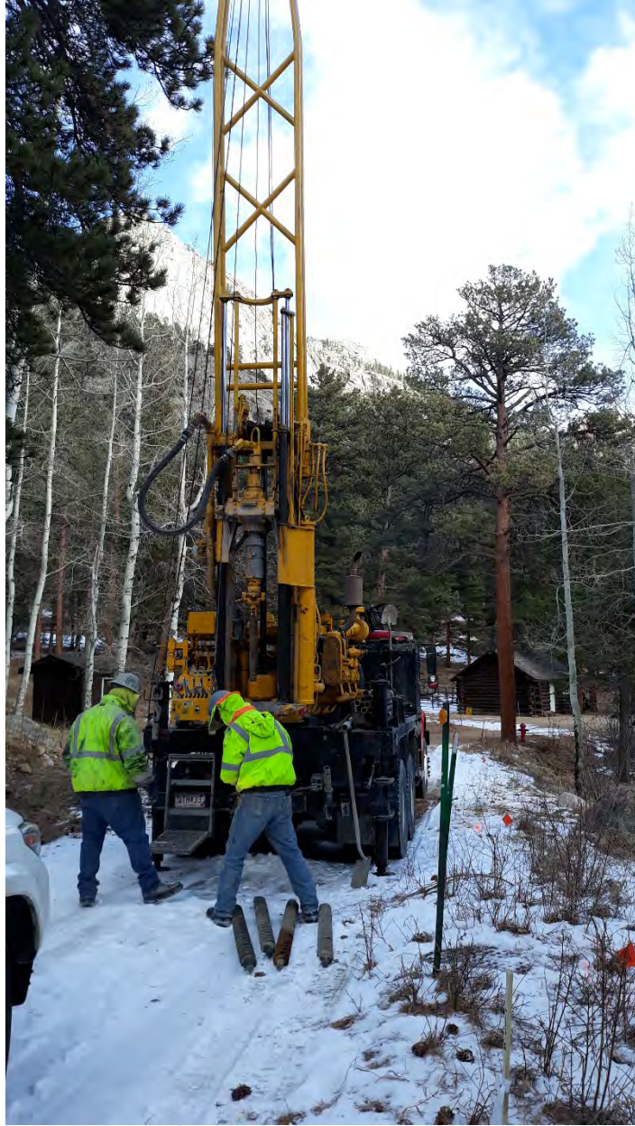
Figure A 6. Drilling boring YA-NW-1.
