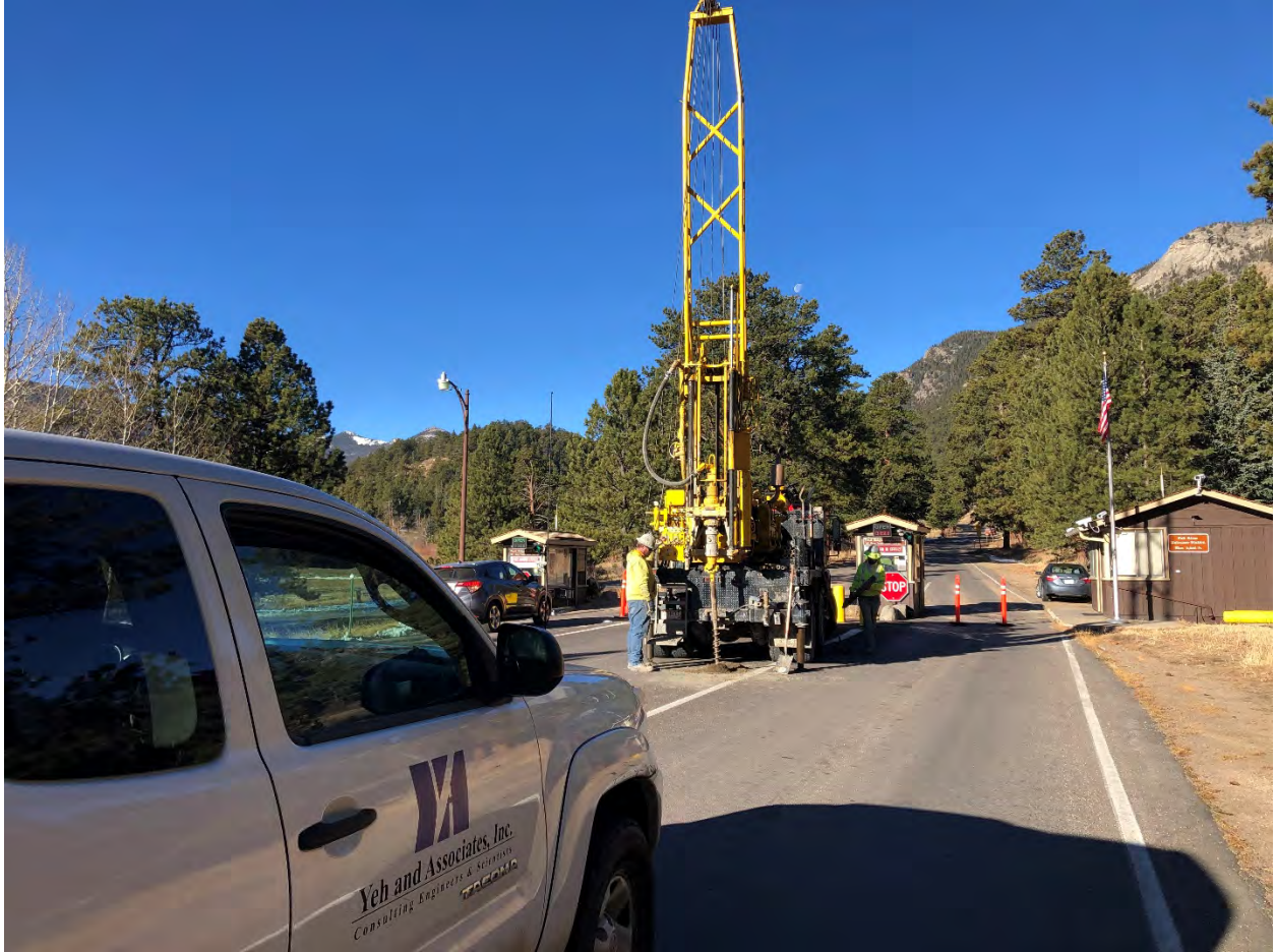
Figure A 7. Drilling boring YA-K1.
